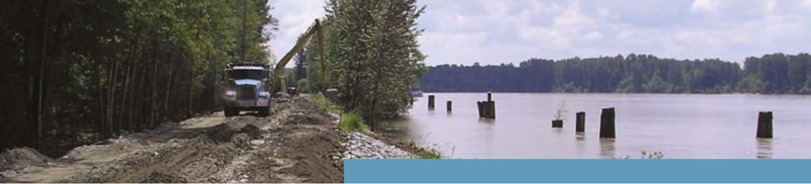
2007 dike upgrades in Maple Ridge. Photo courtesy of District of Maple Ridge.
