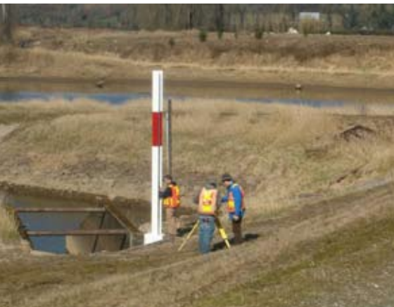
One of 37 new flood warning gauges throughout BC installed by local partners with support from FBC.
