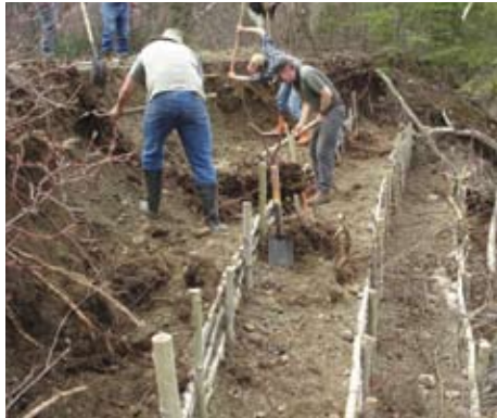
A UNBC student team works on a flood-ravaged site at Naver Creek near Hixon, employing bioengineering techniques for streambank restoration. FBC helped the coordination of several restoration projects.
