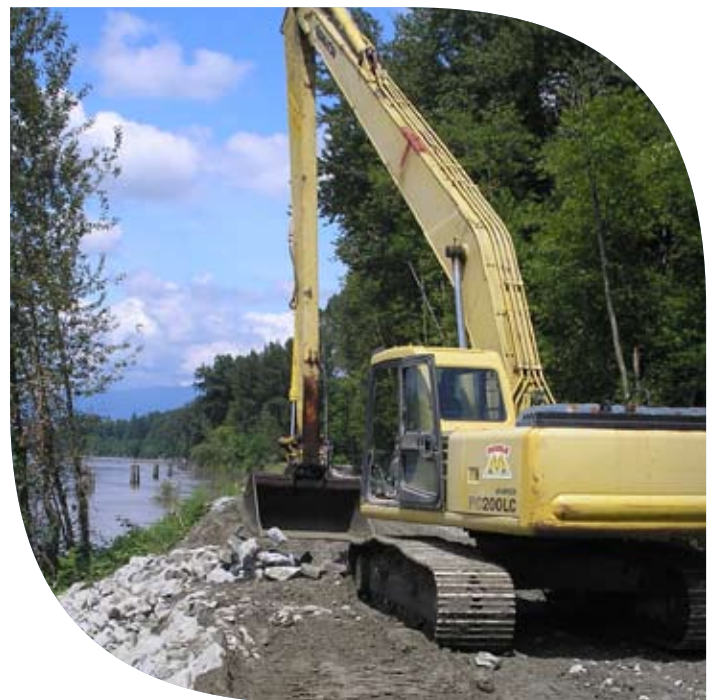
Maple Ridge dike work on the Fraser near Kanaka Creek in 2007. Photo courtesy of the District of Maple Ridge.
