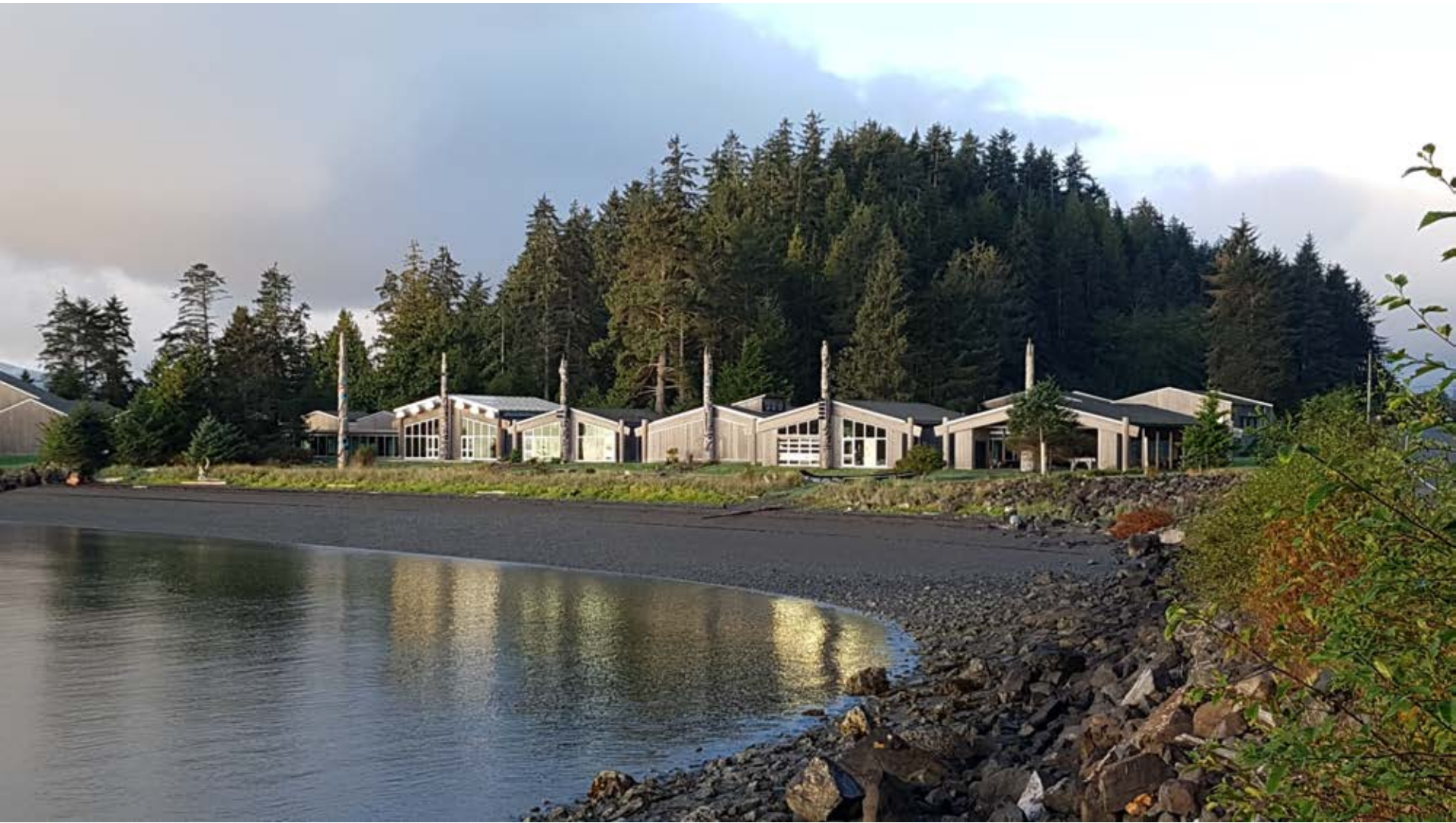
Haida Gwaii- Skidegate 100 kW Solar PV Project
