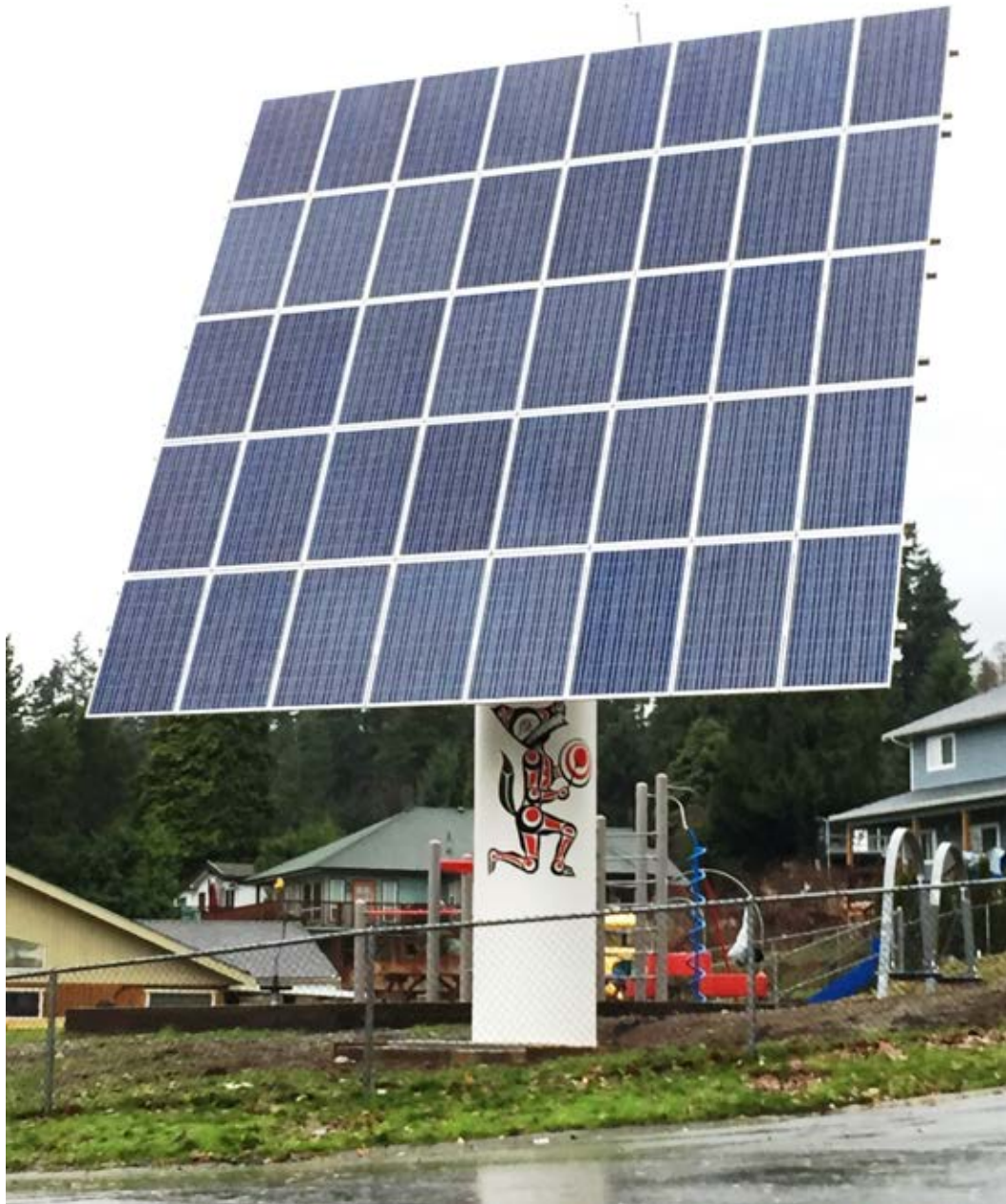
Tsleil-Waututh First Nation 10 kW Solar Tracker
