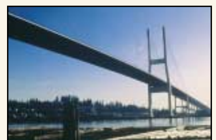
Alex Fraser Bridge
