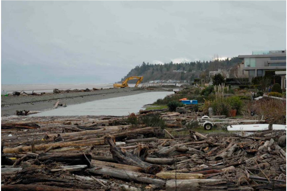
Fig. 7. Damage to shore property after the February 4, 2006 storm in Delta. Source: Corp. of Delta.
