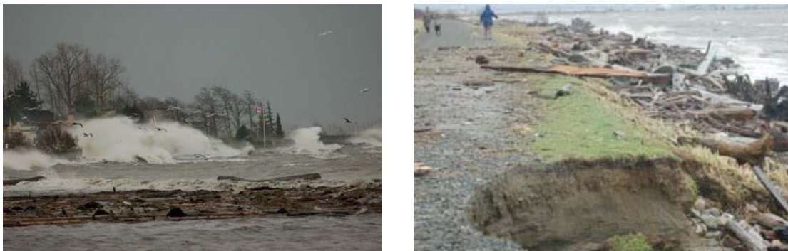
Fig. 6. February 2006 storm and consequential damage done to sea dykes along shore of southern Strait of Georgia . Source: Corporation of Delta.
