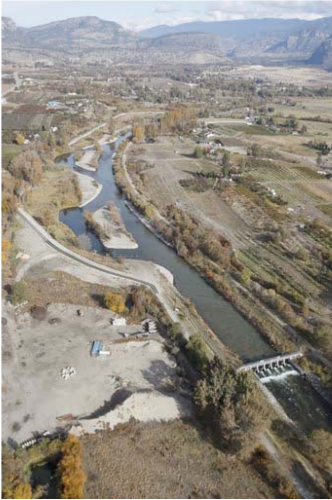
Facing north, the Okanagan River Restoration Initiative is shown on the left side. Photo: Kevin Dunn.
