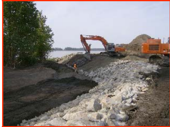
Native sediments placement on riprap
