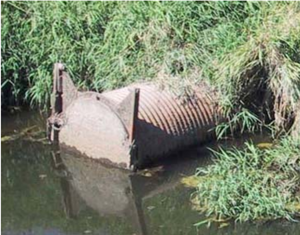
Flood box with a top mounted gate. Photo courtesy of Alan Thomson
