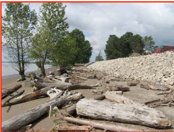
Arrangement of logs at dike toe
