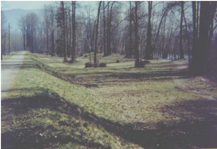
A setback dike with mature vegetation retained in the river corridor. It is also important to retain understory vegetation.
