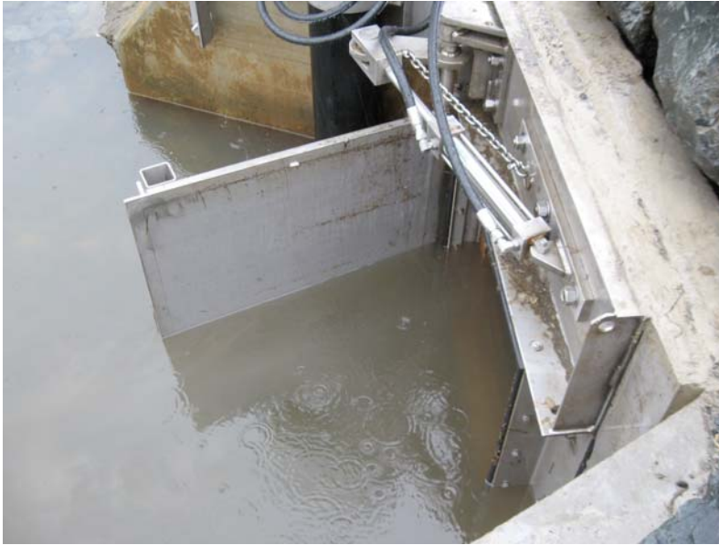
A closer look at the self-regulating tide gate installed in the Nanaimo River estuary. Photo courtesy of Craig Sutherland.
