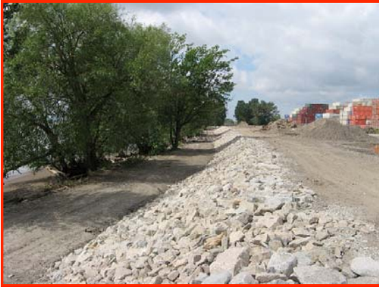
Dike bank protection construction in Richmond
