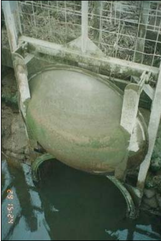
A combination gate (Flap gate and sluice gate combined) is installed in Brown Slough, southeast of La Conner, WA. Photo courtesy of Alan Thomson.
