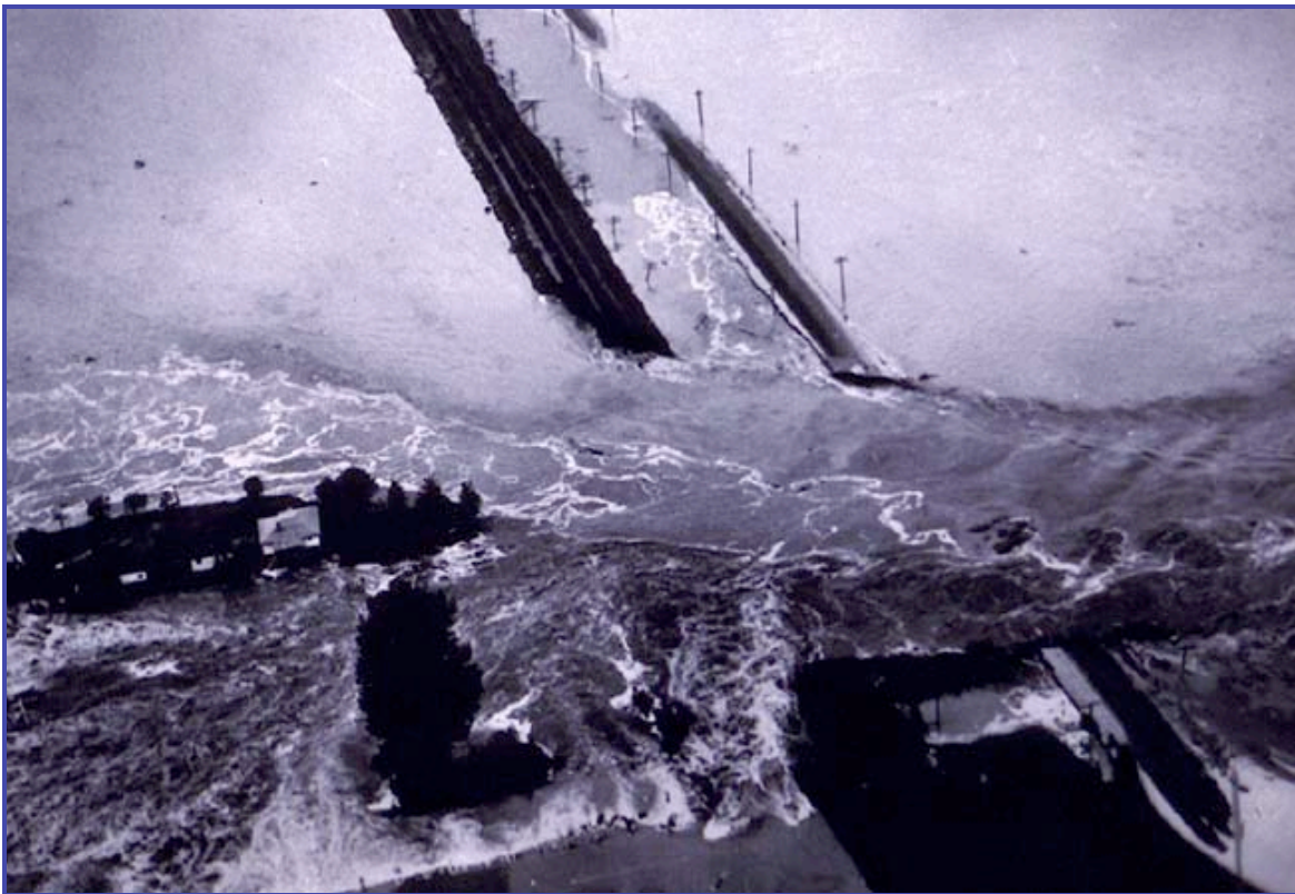
Photo 7 - Dyke break at Hatzic, Fraser River flood, 1948
