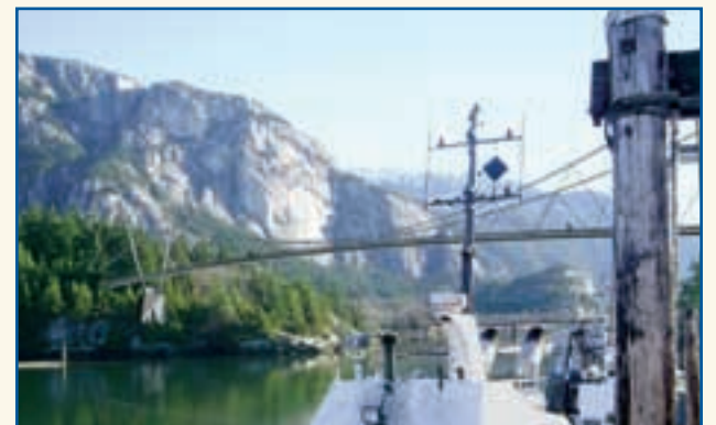
Pedestrian walkway across Mamquam Blind Channel
