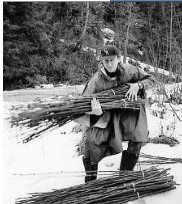
Willow cuttings for streambank restoration activities
