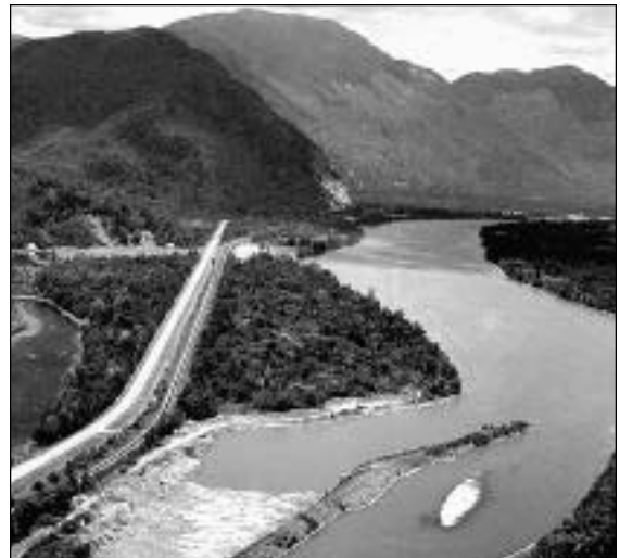
Agassiz Debris Trap: Every year the trap captures enough debris to fill about 10 football fields three metres high.
