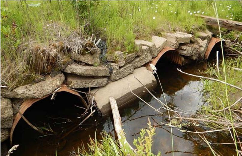
Workshop participants went through a condensed version of the PIEVC Protocol through a small group exercise based on the case study of the McMillan Creek Crossing at Aberdeen Road in Prince George. The structural system includes a precast concrete cap beam, steel pipe piles, a retaining wall and engineering fill. Surrounding utilities includes a 200 mm water main, 900 mm storm main, 450 mm sanitary trunk main, gas main, as well as overhead electrical and telephone cables.
