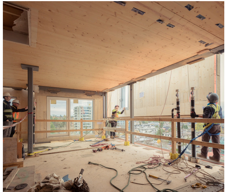
The 81-unit building will feature prefabricated cross-laminated timber floors and Intelligent City's mass timber envelope panels, along with a concrete core and a parkade. Photo: Kristopher Grunert / © Intelligent City
