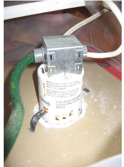
Non-IC-rated air leaky pot-light
