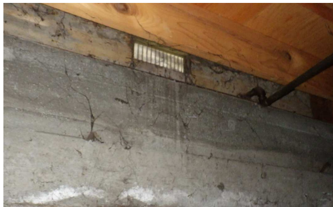
Air vent in the rim joist in an insulated vented crawlspace.
