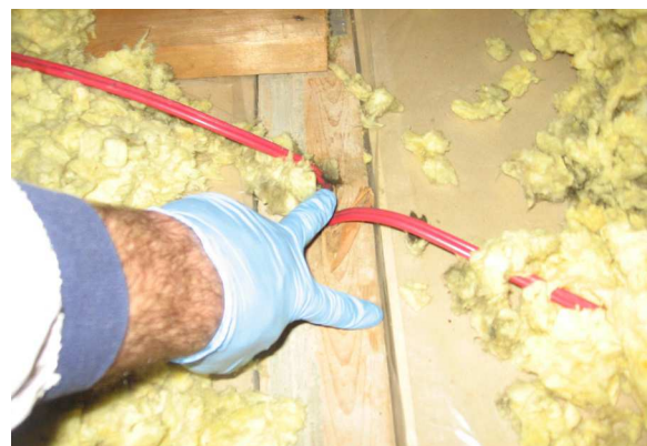
Air sealing of an electrical penetration and unsealed top-plate connection in an attic.
