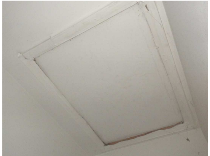
An attic access hatch made from plywood resting on a wood-trimmed opening.
