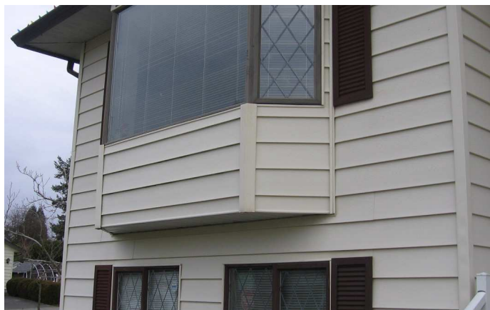
Overhanging floor under a bay window.
