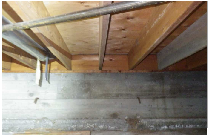
Uninsulated crawlspace interior walls and floor.
