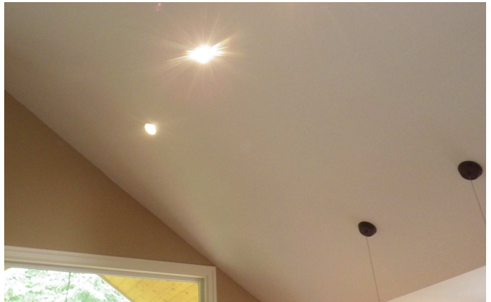
Vaulted gypsum board ceiling with face-mounted and recessed light fixtures.
