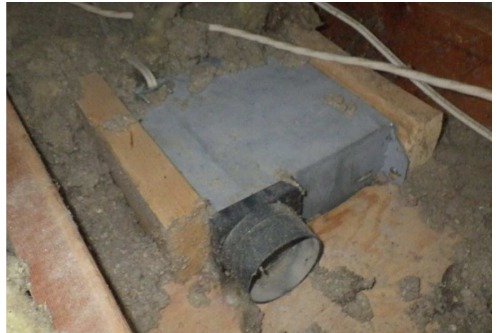
Bathroom exhaust fan venting into the attic. Conditions such as this should be remedied prior to or as part of air sealing and insulation work.
