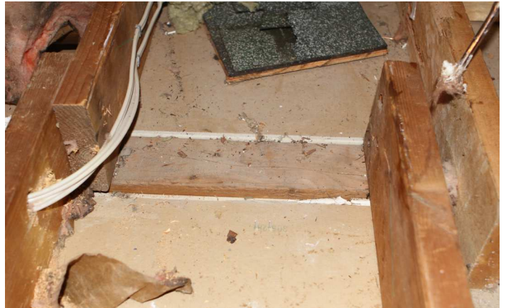
Exposed interior top-plate as viewed from the attic.
