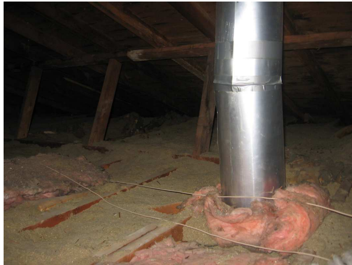
Insulated and sealed exhaust duct in an attic.
