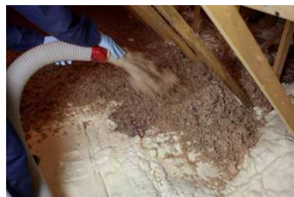
Insulation retrofit of an attic ceiling consisting of blown-in cellulose over top of an air sealing and insulating layer of spray polyurethane foam.
