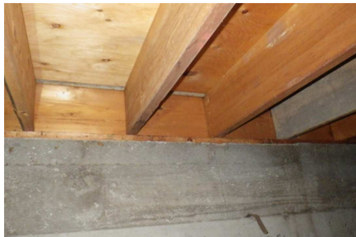
Exposed below-grade wall at floor rim joist.
