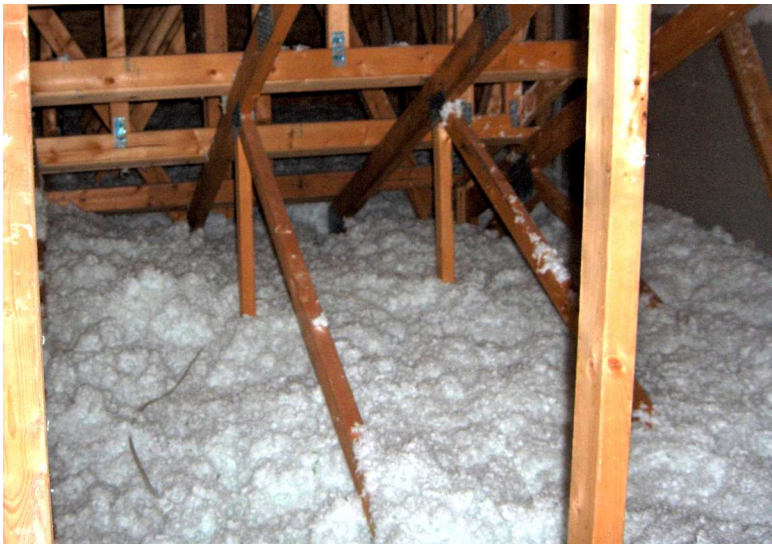
Blown-in fibreglass attic insulation.
