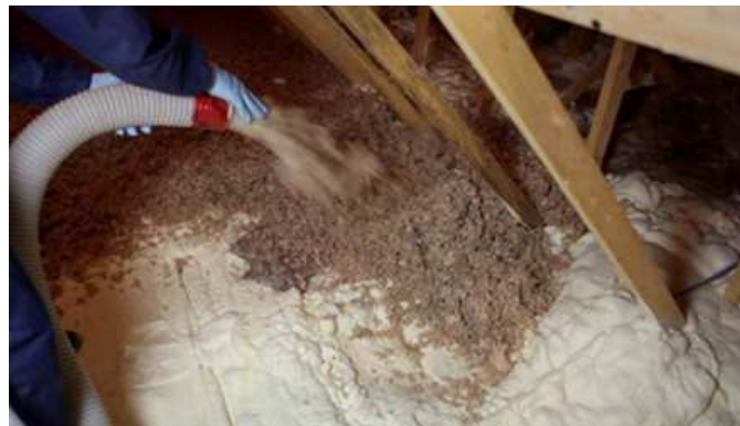
Flash-and-fill attic installation where a few inches of sprayfoam is sprayed to top of ceiling drywall, and then covered with lower cost low-density cellulose or fibreglass insulation fill.
