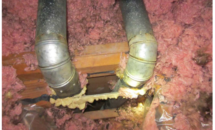
A relatively large hole in the ceiling plane through which two ducts are installed.
