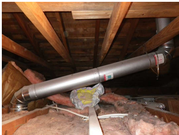
Uninsulated and un-sealed exhaust duct running through attic leaking air and heat to the space.
