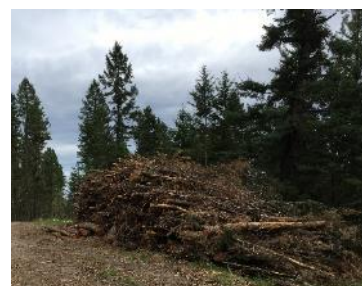
Figure 8: Phases of fuel treatment and timber harvest, WL Community Forest cutblock 106. Falling and sorting was followed by forwarding logs and biomass for delivery to purchasing mills. Timber harvest was combined with debris piling for forwarding, and eventual removal to Atlantic Power.
