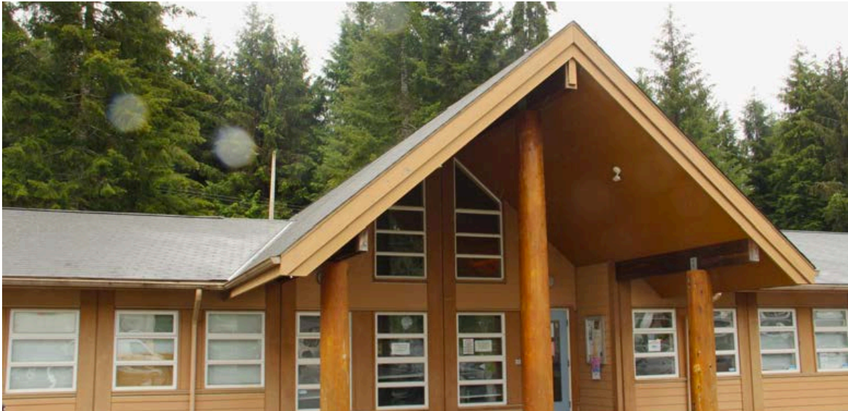
Among Quatsino First Nation's renewable energy projects, a solar power installation for its community building is in development. | Photo credit: Sybil Zhang
