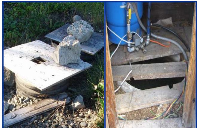
Figure 5: Improperly covered wells
