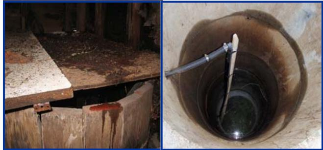
Figure 8: Water able to seep into well through the casing
