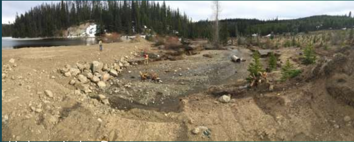
Helmer Lake Dam
