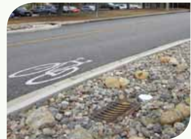
Photos: (Top) Vegetated and (Bottom) un-vegetated rain gardens in streetscapes, City of North Vancouver.
