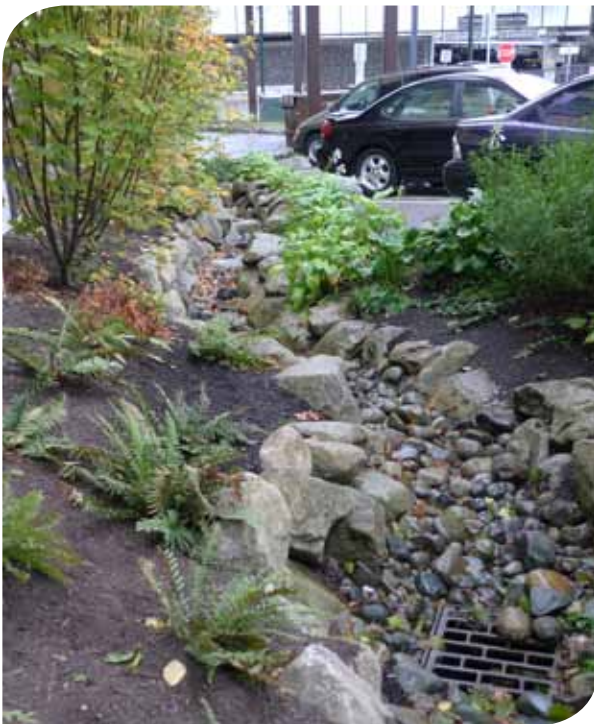
Rain garden on an institutional property captures and infiltrates runoff from adjacent parking lot and other impervious surfaces.
