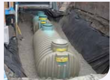
Photos: (Top) Green roof and (Bottom) underground cisterns at UBCM Local Government House in Victoria, BC.
