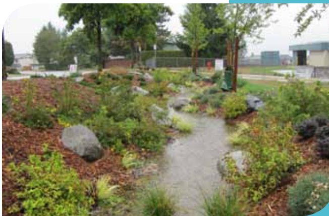
Completed rain garden captures and infiltrates runoff from nearby impervious surfaces, Brook Elementary, North Delta, BC.
