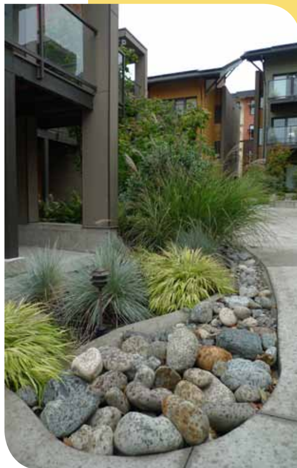
Rain garden in a multi-family residential community infiltrates and cleans stormwater collected from surrounding impermeable surfaces.
