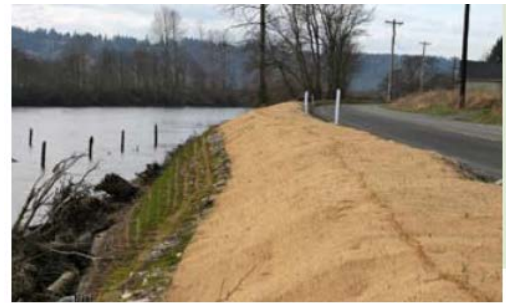
Eventually the coir fabric and the structural earth wall itself will be completely overgrown with hydro-seeded grass and other vegetation.
