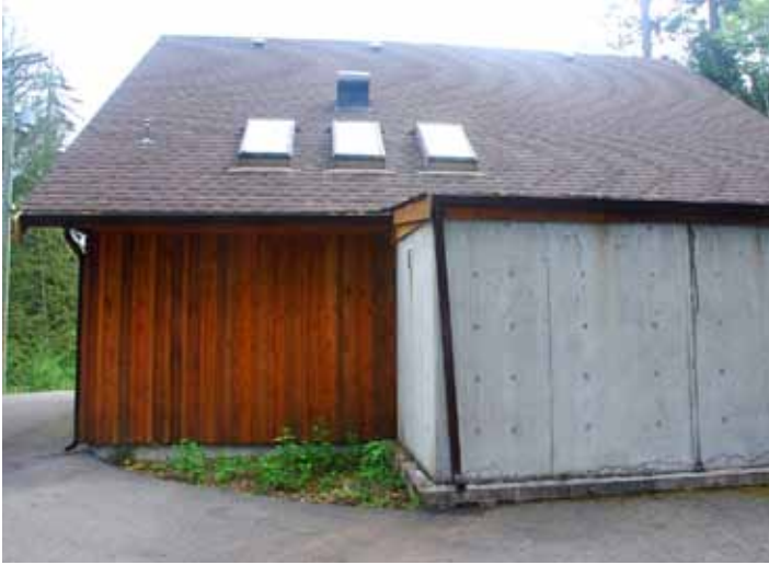
The well-kept Nanoose station replaced the old failing septic systems with collection pipes, a pump station, the treatment facility and 2.2 km ocean outfall. photo by Denise Hoskins
